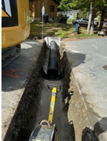
Diagonal Cross Culvert on Fauxburg Road
