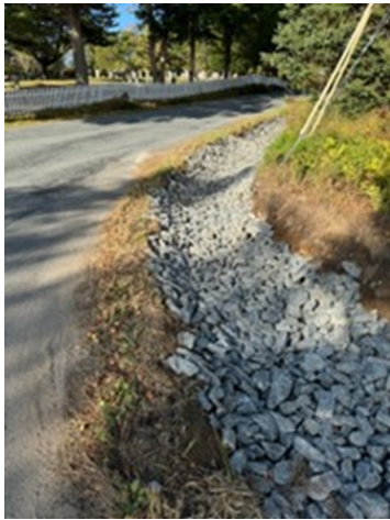
Ditching and Armouring on Clearland Road
