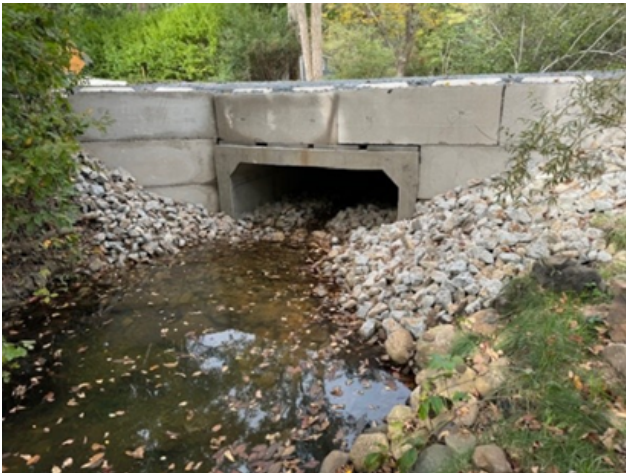
New Box Culvert on Wye Street
